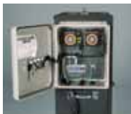
Timers are located in a water-resistant control panel and automatically provide aeration and microbial injection.
